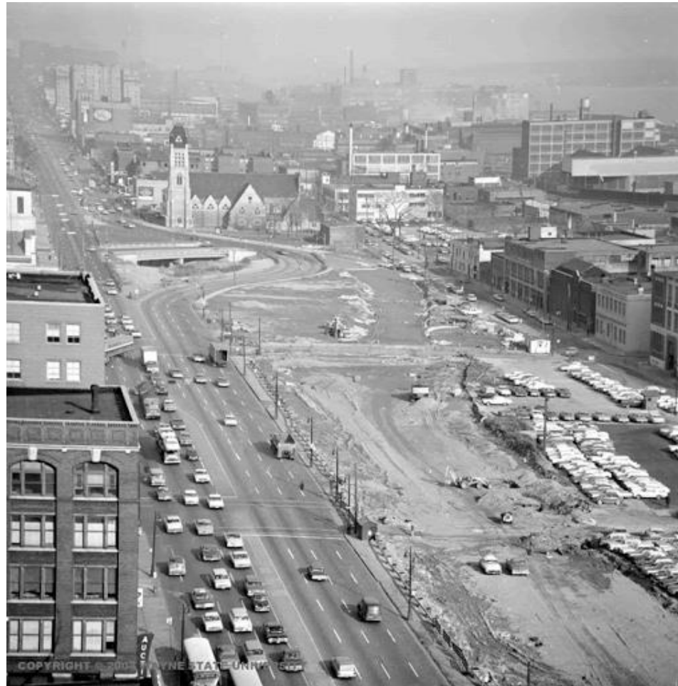
Chrysler Freeway construction in Detroit, MI
